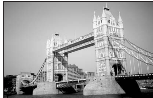
Tower Bridge, London, England.
